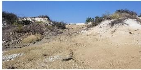
ID:1 Erosion: 94.40 Mg ha -1 yr -1 , SOC: 1.58 Mg ha -1 Land use: Bare Soil Practice: None Easting 662949 m, Northing 1964523 m, Photography taken westward.
