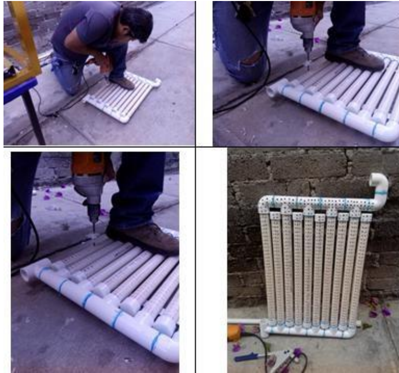
Figura 13 Pipes for dehydrated air recirculation
