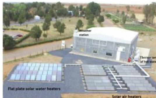
**Figure 1-11.** Solar pilot plant for drying agricultural products (García-Valladares et al., 2020).
