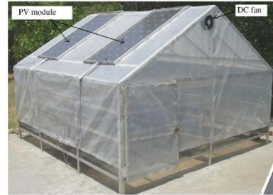
**Figure 1-8.** Greenhouse-type solar dryer with plastic cover and Venlo geometry (Barnwal & Tiwari, 2008a).
