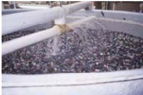
Fig. 2.10. Rock packed bed biofilter.
