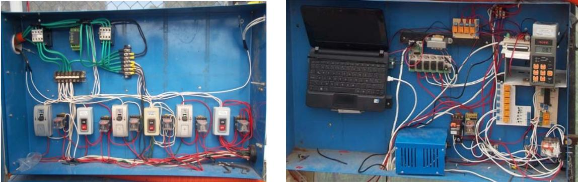
Fig. 3.32. A central controller PC for dissolved oxygen controller with dissolved oxygen analyzer (HI 8410).
